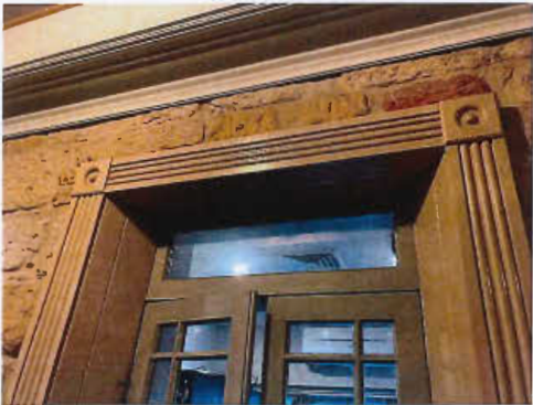
Figure 23 – Detail of door architraves
