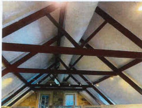
Figure 28 – Timber trusses in attic
