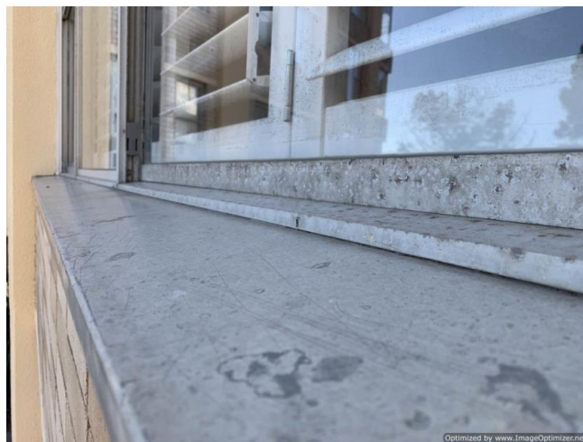
P1 – oxidisation of frames due weathering
