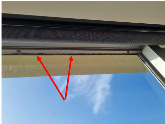
P3 – Putty around the window has deteriorated
