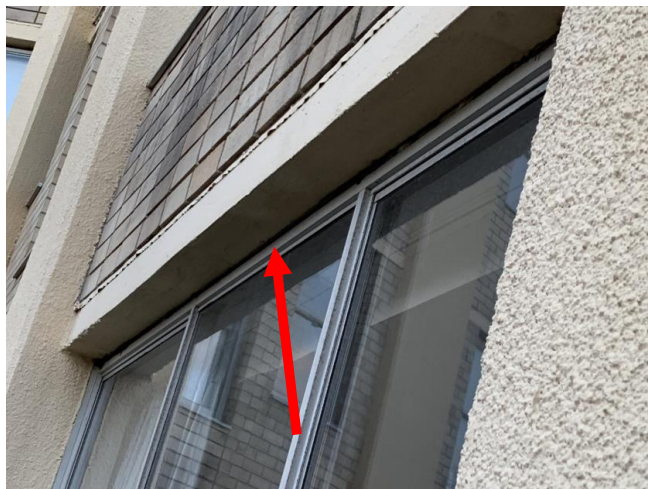
P4 – deteriorated sealant at head of window
