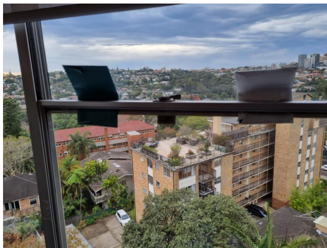
P2 – Paper inserted between window sashes to prevent rattling
