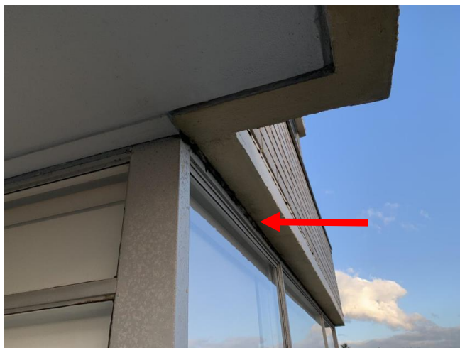
P5 – oxidisation and failure of sealants around window frame
