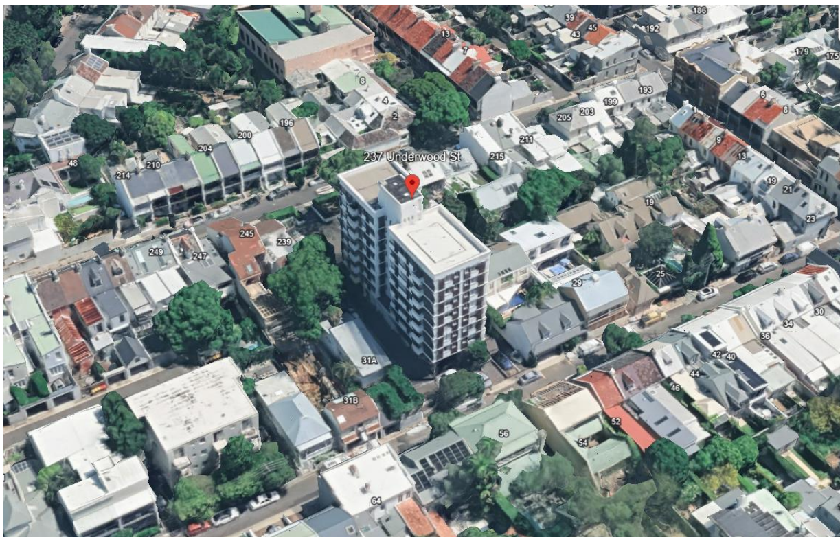
Figure 1 – 3D View to the subject site and demonstrating the context (Source: Google earth)
