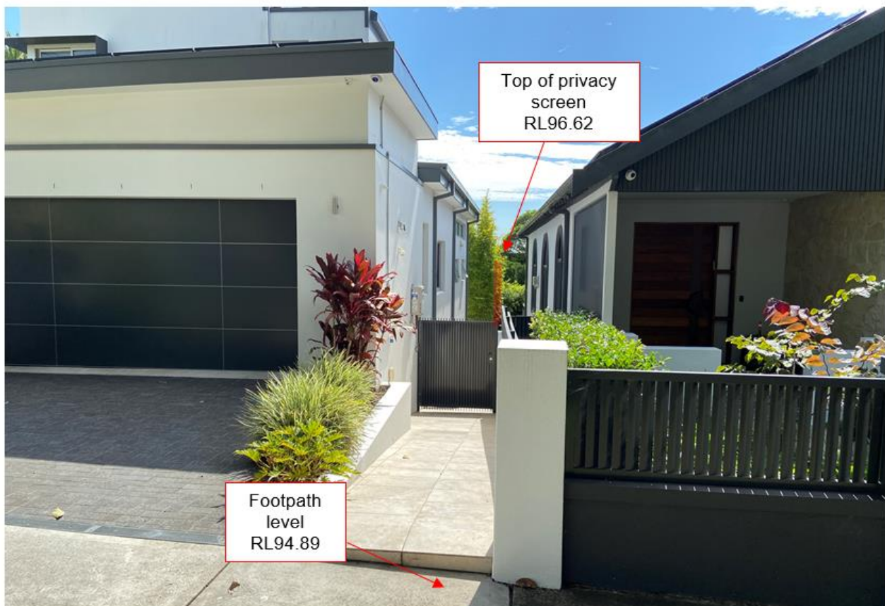
Image 8: View of the existing side boundary showing the approximate location of the new privacy screen, viewed from the footpath level. Source: Original Assessment Report DA27/2024/1
