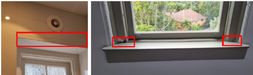
Figure 24 Tiles and timber window frame
