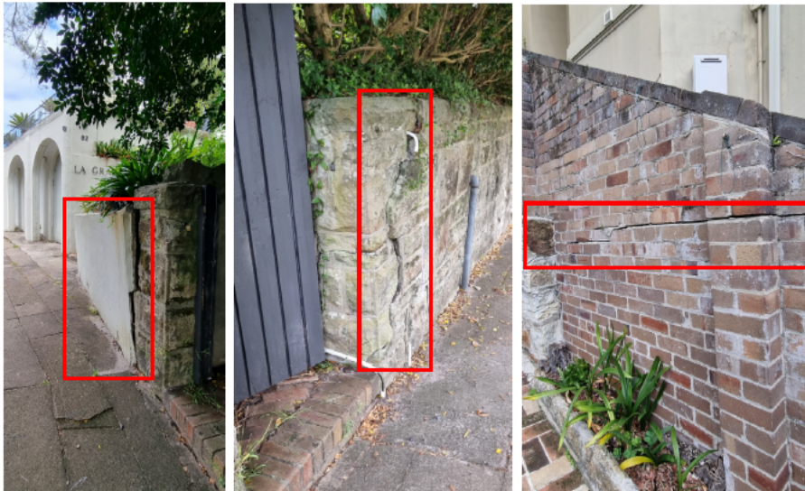
Figure 22 Brick/block retaining walls
