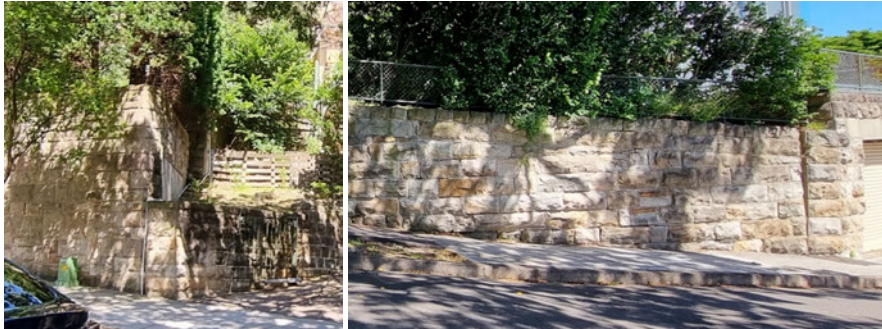
Figure 19 Sandstone block retaining walls
