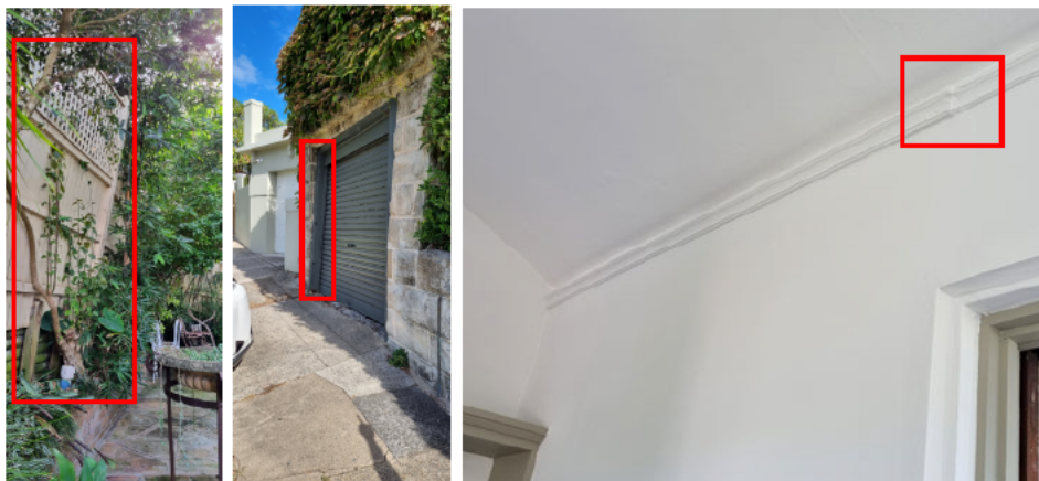
Figure 25 Timber fence and garage door
