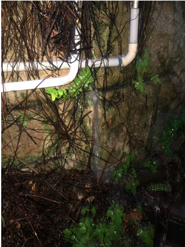
Figure 5 – Photograph of uncontrolled stormwater discharging through the retaining wall
