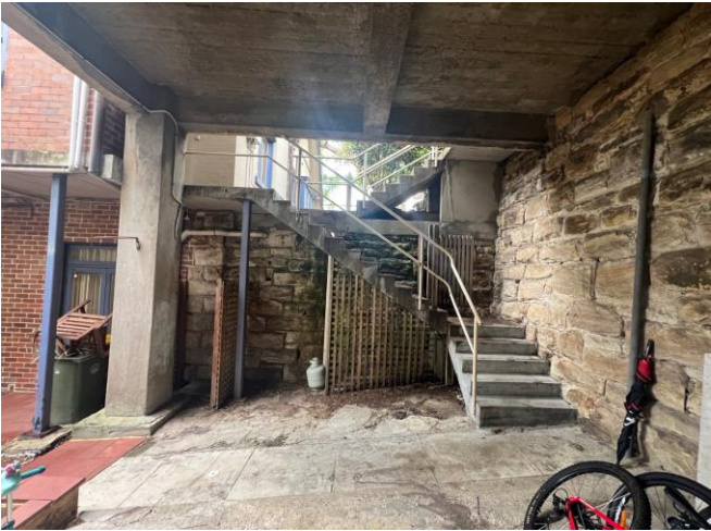
Area below existing raised garage structure with existing sandstone retaining walls
