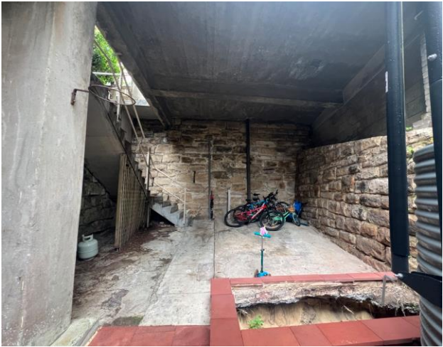
Area below existing raised garage structure with existing sandstone retaining walls
