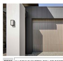
EF09 ALUMINIUM BATTEN ROLLER DOOR Colour - to match EF07 or similar approved
