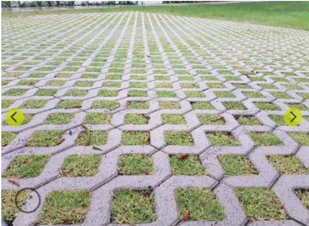
Figure 8. Example of “concrete grass diamond paver” provided by the Applicant. Source: Submitted Additional Information
