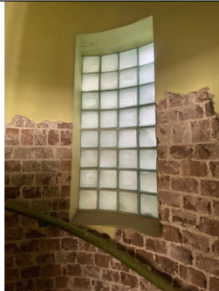
Figure 14. Glass brick window in stairwell, characteristic of geometric fashions in the interwar period.
