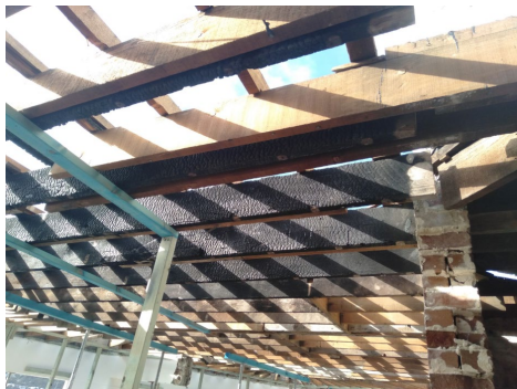
Figure 4.26 Ceiling rafters with areas of burnt rafters exposed. (Source: GML, July 2024)
