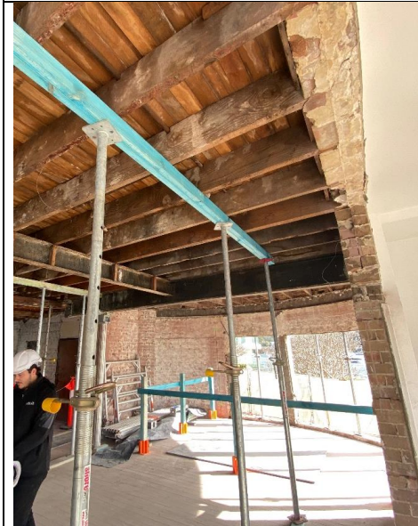
Figure 13. Original timber and steel floor structures and decking. (Source: GML, August 2024)
