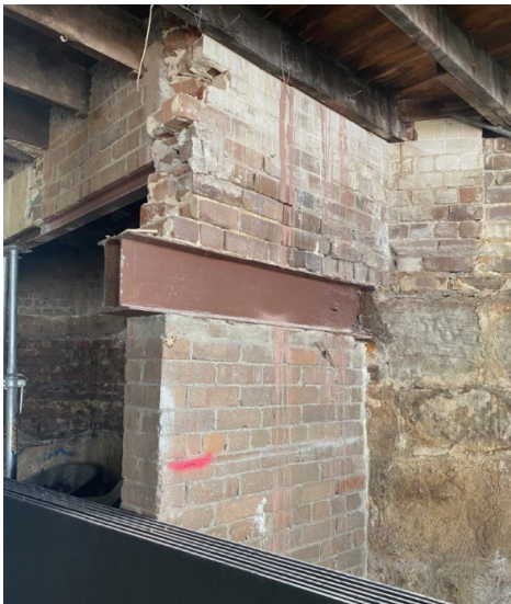
Figure 4.20 Severed beam in basement. (Source: GML, July 2024)
