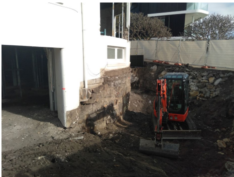
Figure 4.18 Excavation in front of the northwest elevation, revealing sandstone foundations. (Source: GML, July 2024)
