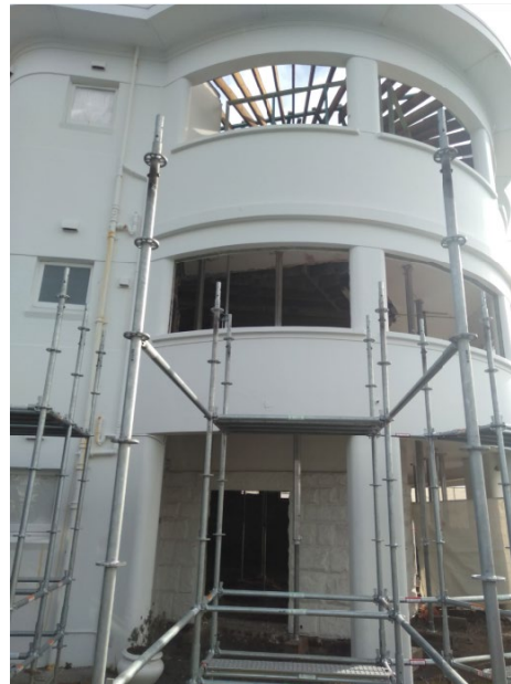
Figure 4.17 Eastern elevation of dwelling showing 1916 sandstone basement wall (painted white) and form of 1939 addition above. (Source: GML, July 2024)
