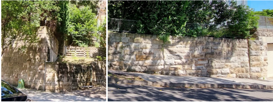
Figure 19 Sandstone block retaining walls
