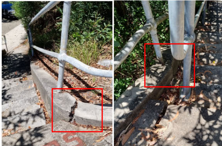
Figure 18 Cracked hand-rail kerb along an external stair.
