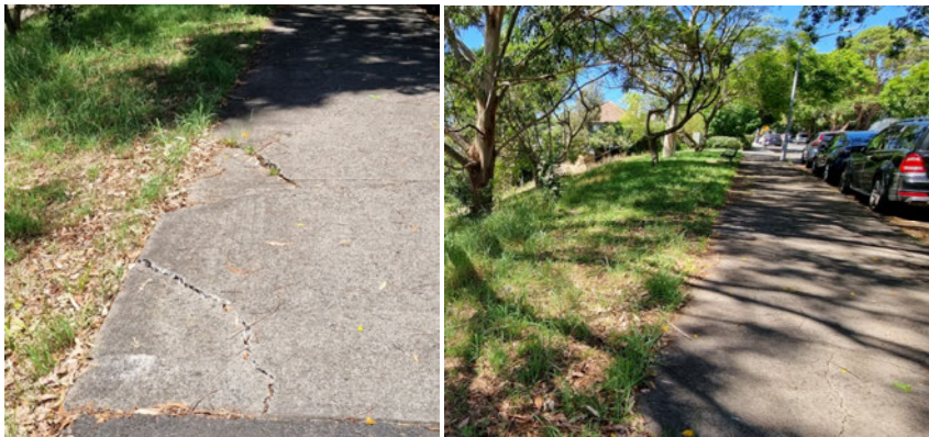
Figure 16 Tension cracks on footpath along Cranbrook Road
