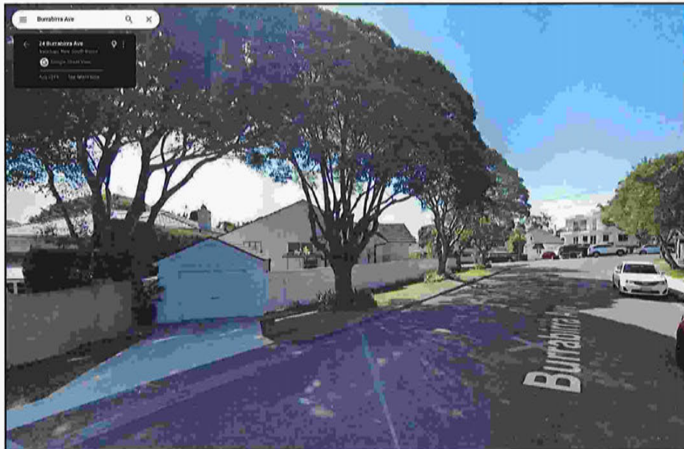
Google view of garage of No 14 Fitzwilliam Rd: No gutter drains and no driveway kerb lip are present
