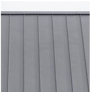
Zinc Standing Seam Roof
