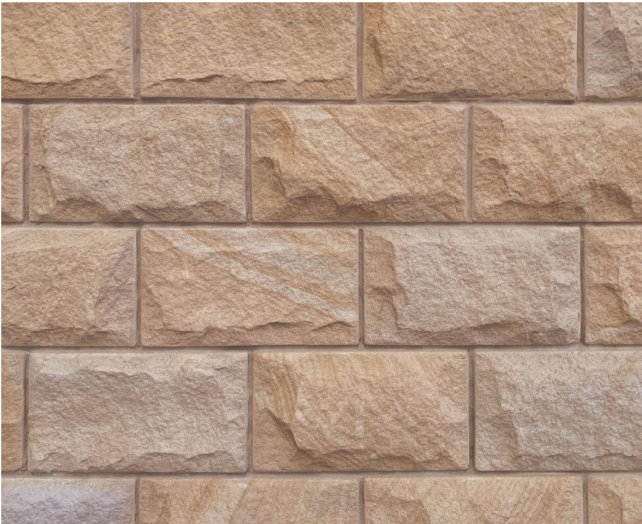
SANDSTONE ASHLAR BLOCKS TO EXTERNAL LOWER GROUND FLOOR FACADE
