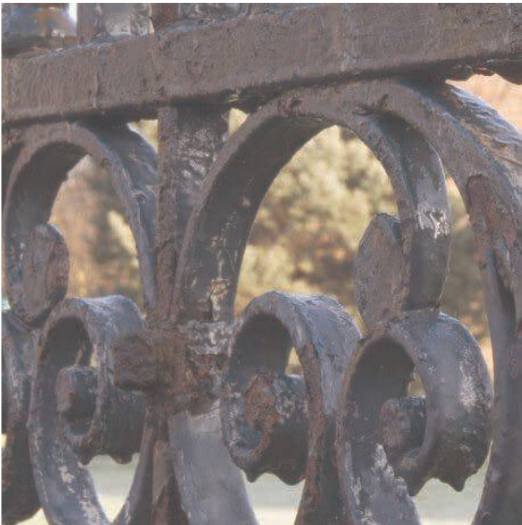
WROUGHT IRON (BLACK PAINT FINISH) BALUSTRADES
