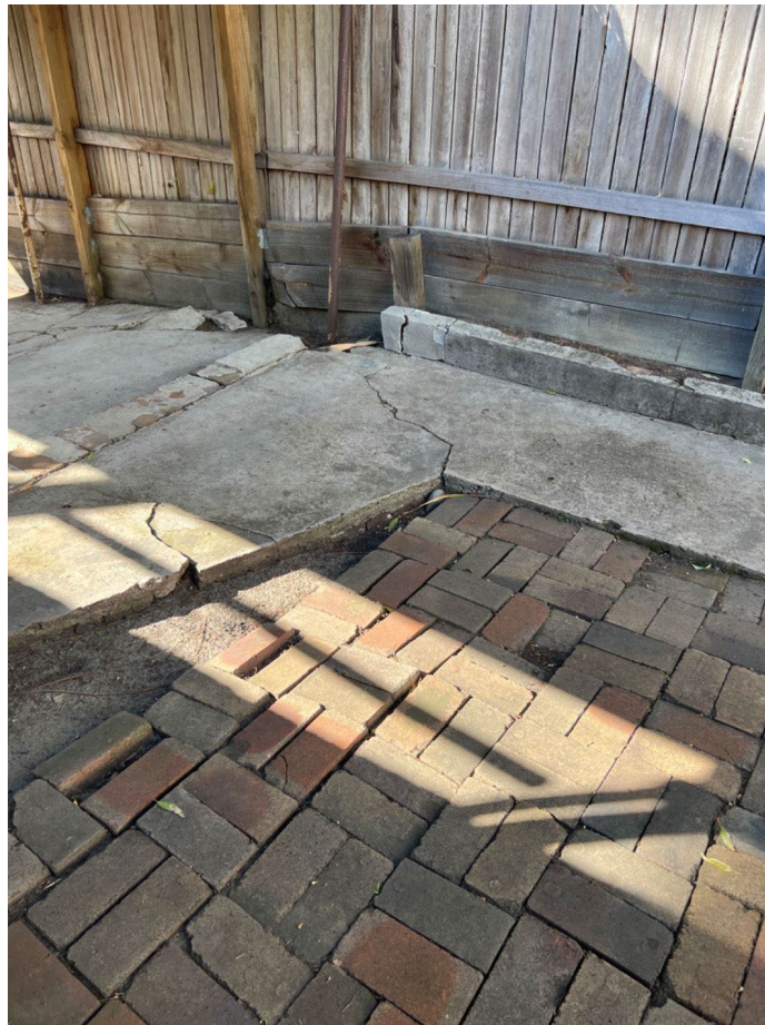
Figure 3 - Localised radial deformation of paving and retaining wall, indicating surface structural roots.
