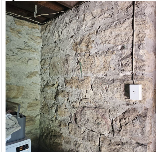
Figure 9: Lower Ground, sandstone basement walls, this wall to be demolished.
