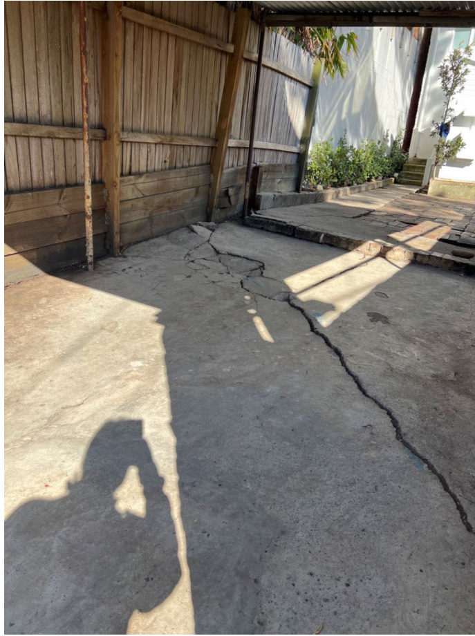
Figure 2 - Radial deformation and cracking of concrete indicating surface roots
