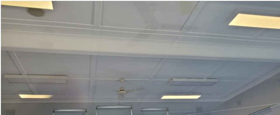
Ceiling of classroom on the second floor with ceiling joists and baton detailing (Artefact, 2023)
