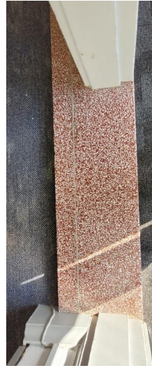
Terrazzo threshold at entrance to classroom from corridor, also showing timber doorway and skirting board. The terrazzo is a further indication that this was originally an external doorway to an unenclosed verandah (Artefact, 2023)
