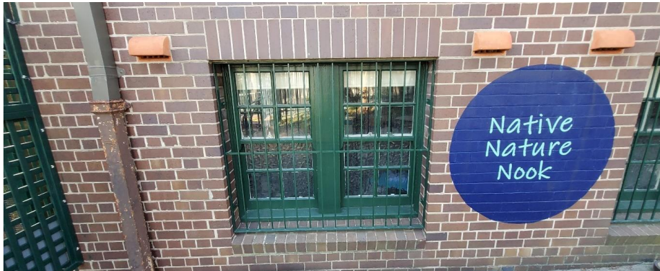
Detail of metal windows with security bars, brickwork and downpipe on façade facing Carlisle Street, with painting promoting a school activity over the face-brick surface (Artefact, 2023)
