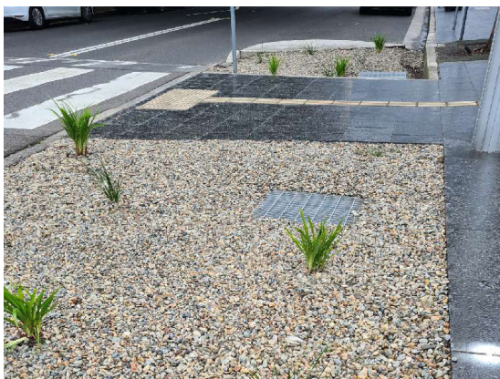
Raingarden installation at pedestrian crossing
