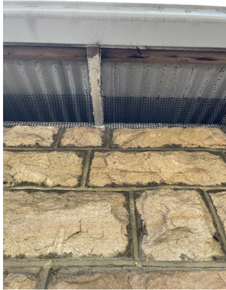
Figure 21: A close up view of concrete pointing to west façade. (Source: Author)
