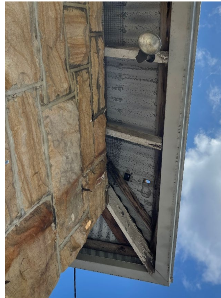
Figure 22: Water damage to timber trusses, and damaged corrugated roof sheeting at the south-east corner of the garage. (Source: Author)
