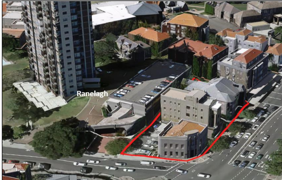
Figure 1: 3D view of site (highlighted in red) from the west (source: Woollahra Council Maps).
