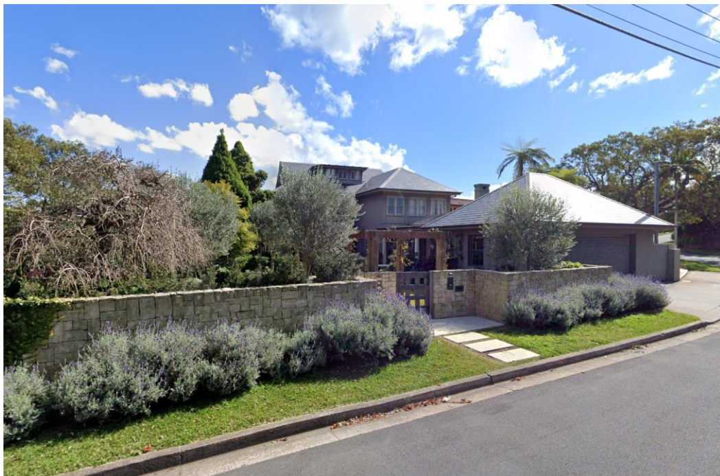
8 Fisher Avenue street frontage
